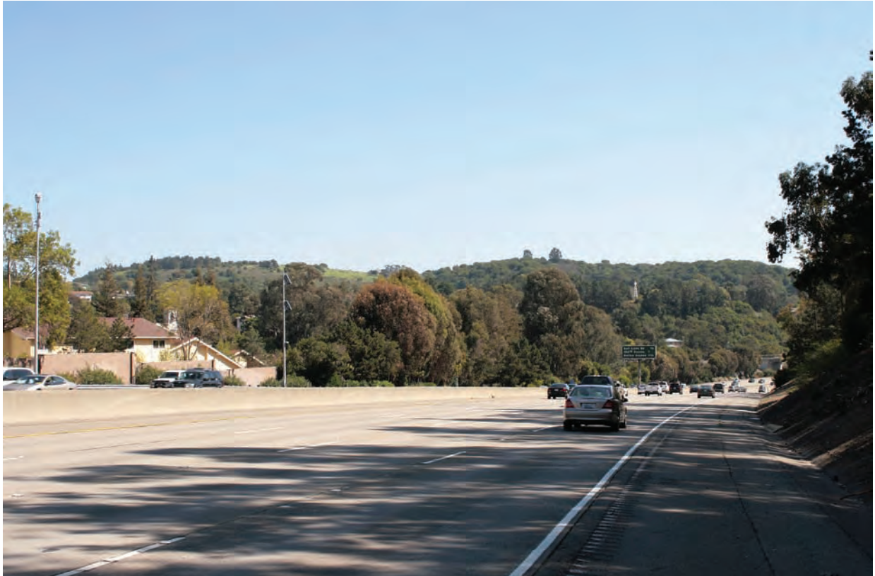
Existing view from I-580 looking south
