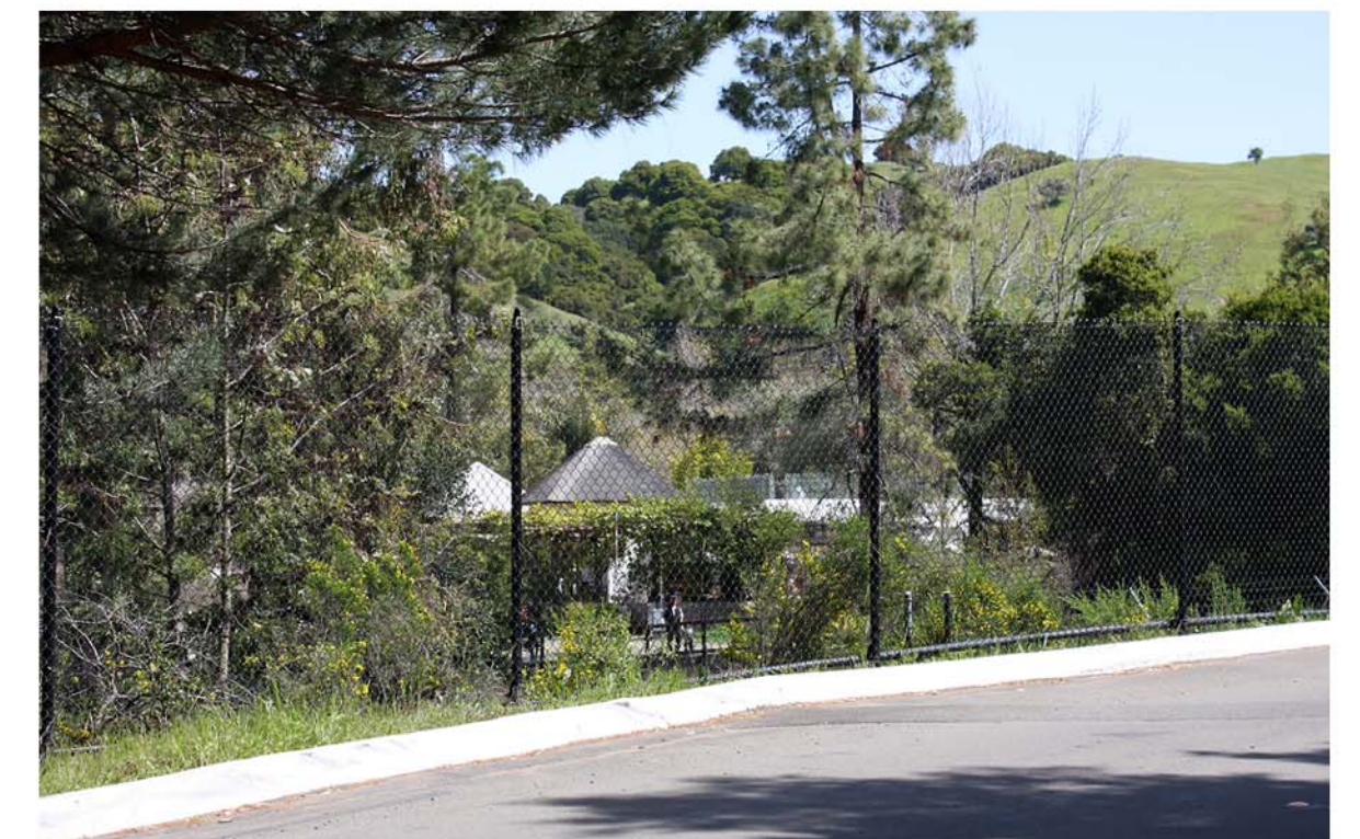
Perimeter Fence TYPICAL REPRESENTATIVE IMAGE OF PERIMETER FENCE
