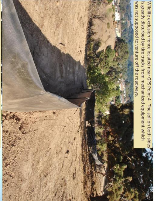
equipment. Permit specifies that mechanized equipment is not allowed Wildlife exclusion fence in fragile native grassland near GPS Point 4 to venture off roadways in this area. reveals greatly disturbed soil due to tire tracks from mechanized
